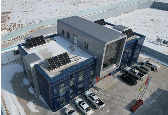
Chicheng Guohua Cadmium Telluride BIPV Curtain Wall Project
