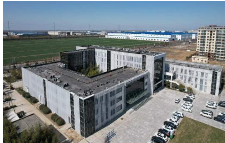
Yancheng Dafeng Yangtze River Delta Wind Power Industrial Park Project
